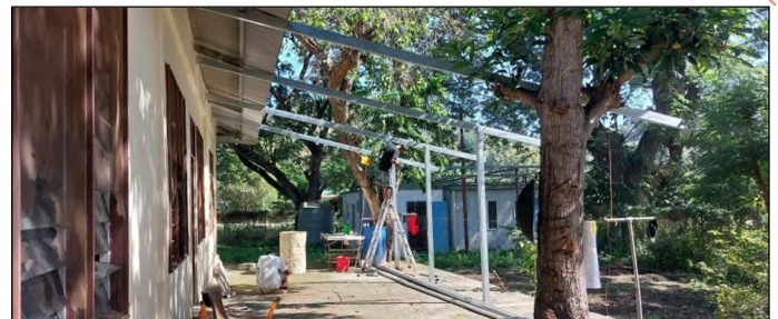
The construction of a tin roof to create the annexe at the back of Uma Garton.
